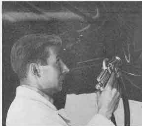
A modern vehicle being treated with B.M.C. Underbody Seal. Underbody Seal is the finest rust preventative and is easy for the operator to handle. Areas recommended for treatment include underbody chassis, underside of wings, inside door panels, and battery boxes.
